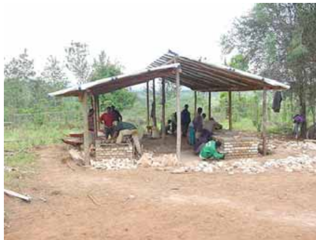
Burundi 2001, roofing allowing smoke to escape.
